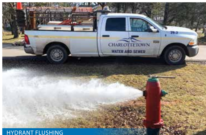
HYDRANT FLUSHING
